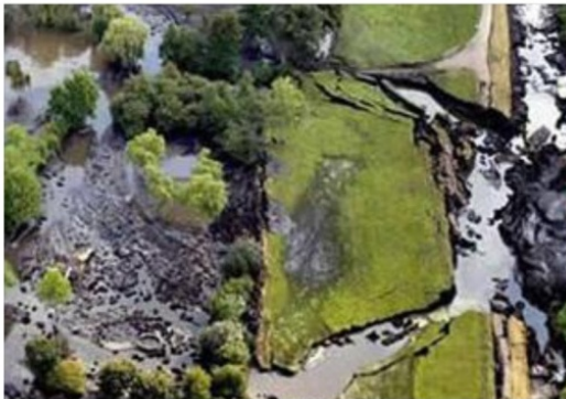
Levee breakthrough (drought)
